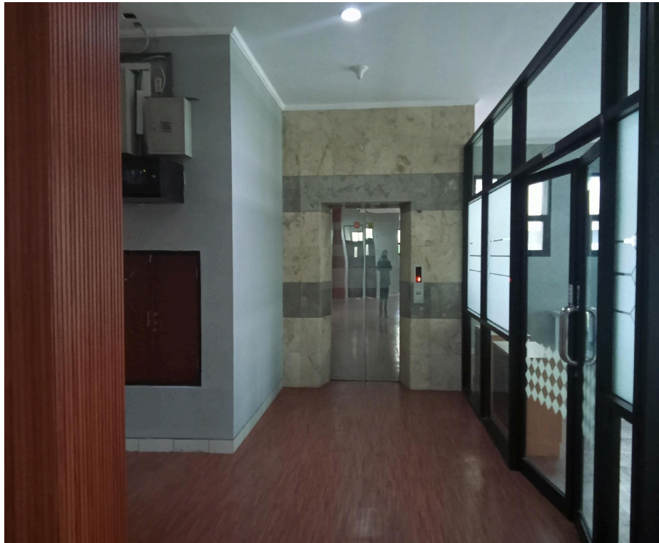
Gambar lift Gedung C
